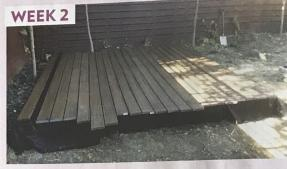
THE DECKING boards are laid in place before being fixed and cut into shape.
