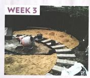
THE SETTS OF THE PATH go down first, while a layer of compacted sand forms a smooth underlay for the lawn.
