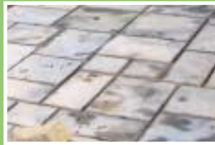
The slabs mortared onto hard core
