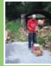
The base is tamped down level
