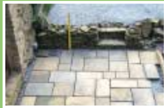
Slabs laid roughly into position
