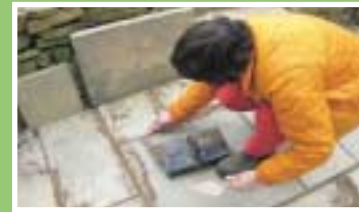
A dry mortar mix is applied to gaps
