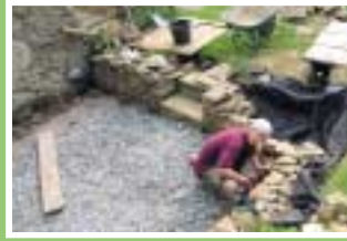
Hard core is laid over drainage
